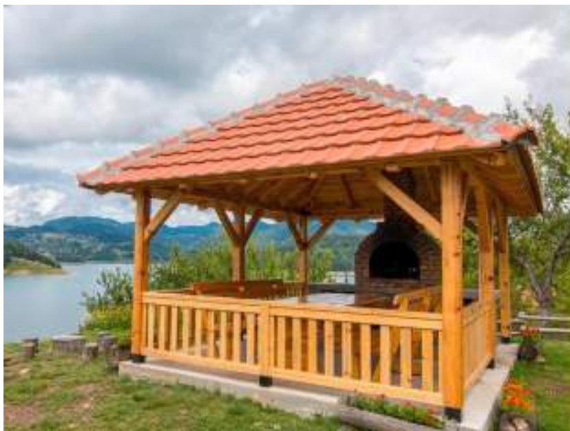
Picture 2: gazebo made of stone slabs, wooden construction and covered with clay shingle- (without designated barbecue)
